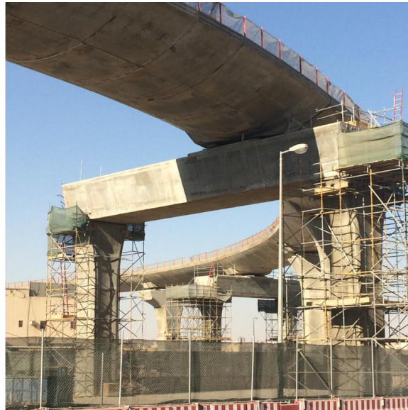
Figure 10 – Construcion of C-Pier & Straddle Piers
