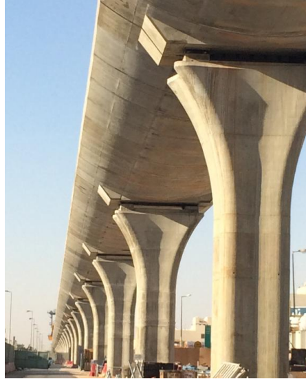
Figure 9 – Basic Pier Shape
