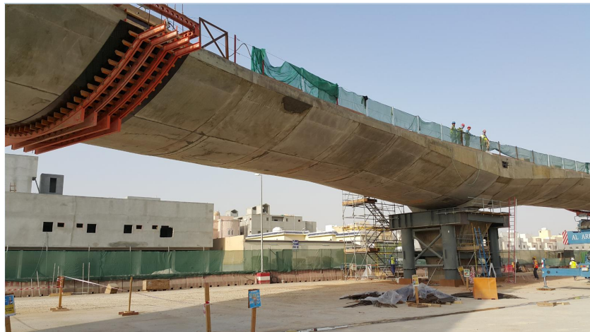
Figure 8 – BCC closure joint construction
