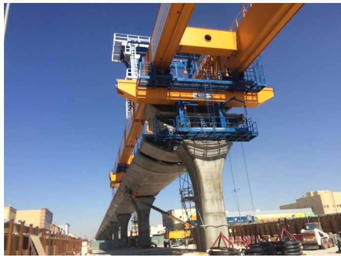
Figure 7 – LG erecting SBS span
