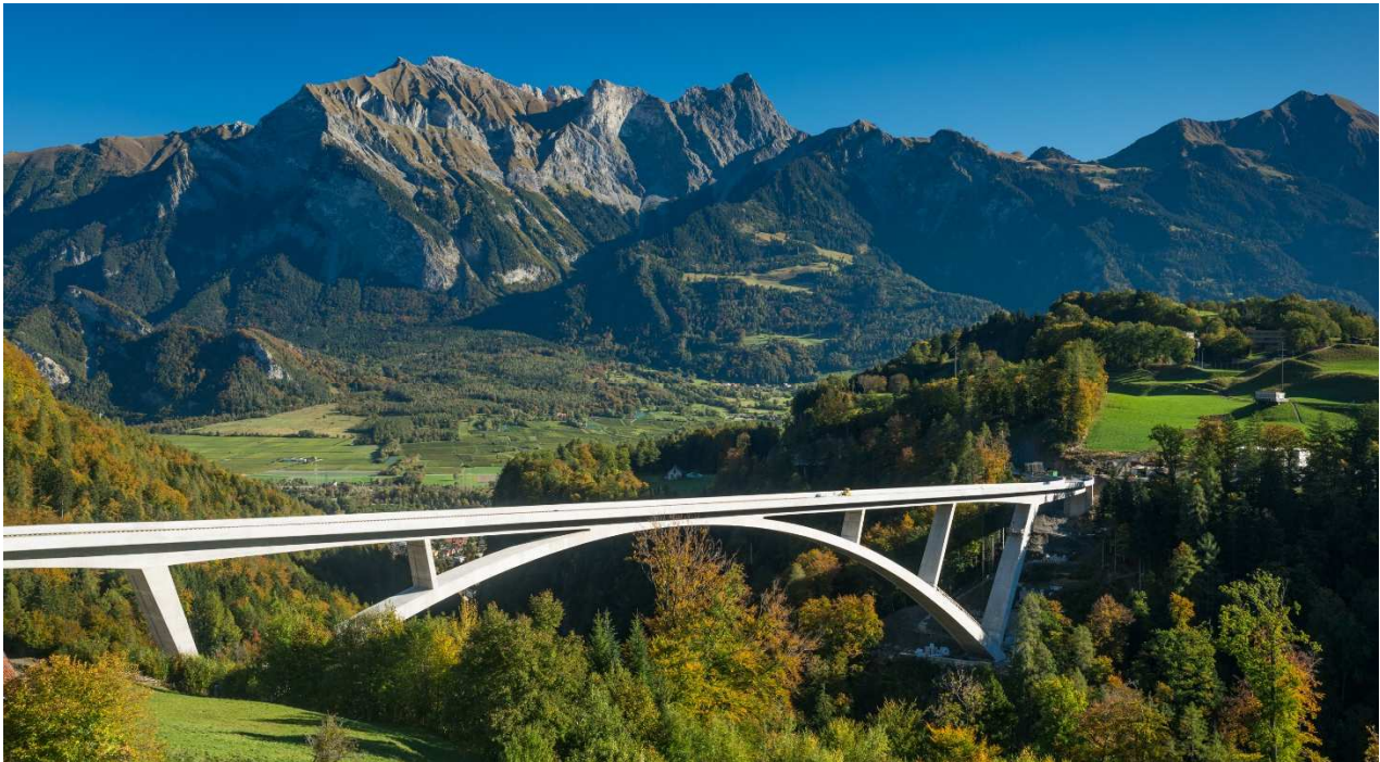
Figure 3. Tamina Arch-Bridge, View from West, © Bastian Kratzke
