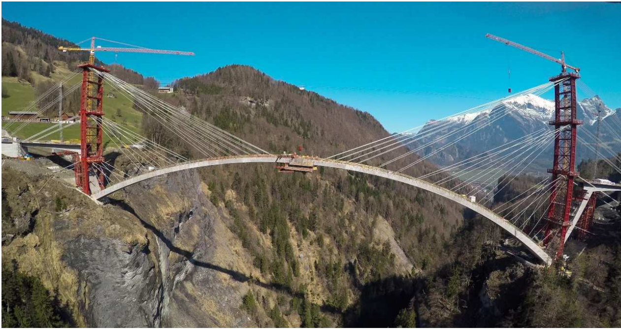
Figure 7. Erection of arch as free cantilever
