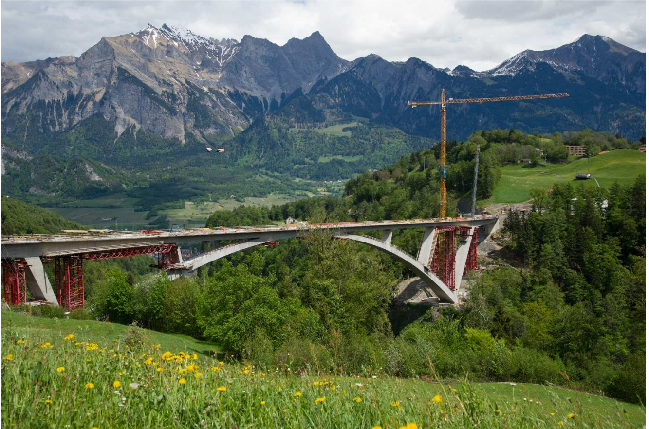
Figure 9. Falswork construction
