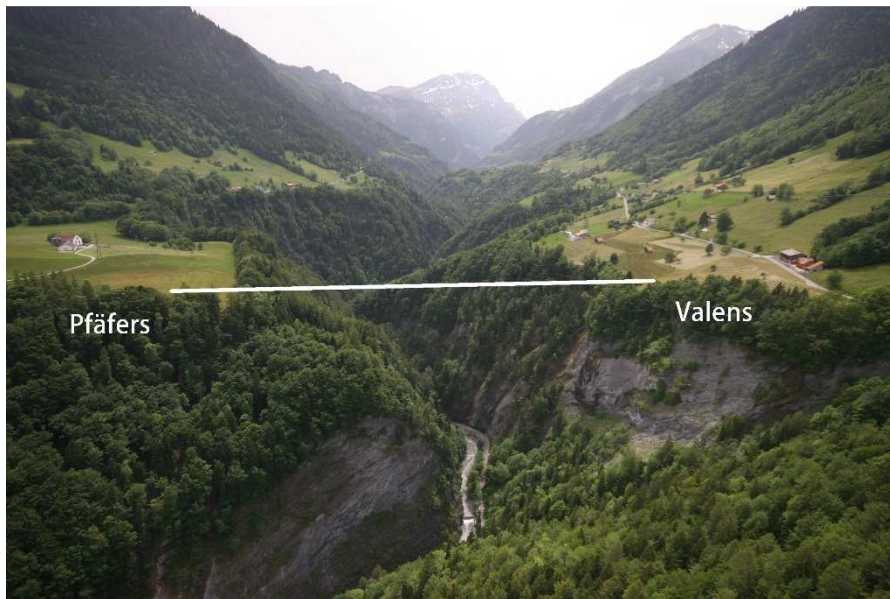
Figure 1. Tamina Bridge, View North-West © Tiefbauamt St. Gallen
